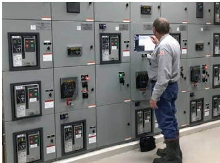
Paralleling Switchgear
